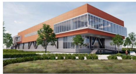
(b) Data center, Irvine, California
