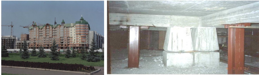
Figure 5 Building on kinematic supports in Novokuznetsk
