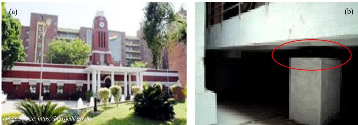
Figure 12 (a) LNJP Hospital Structure and (b) Installed Base-Isolator Unit in the Hospital Structure
