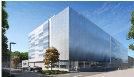
(a) Data center, Santa Clara, California
