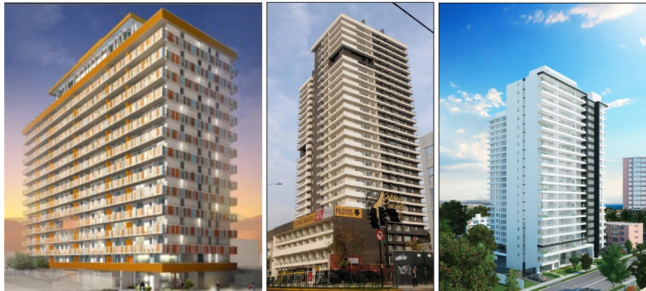
Figure 8 Examples of seismically isolated tall residential buildings in Chile: Torre del Sol (left); Nunoa Capital (center); and Via Poniente (right)
