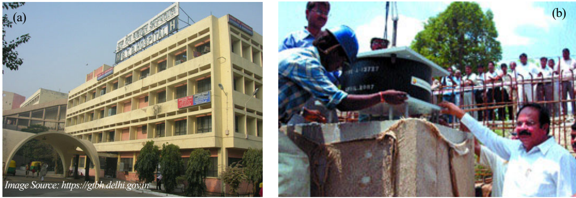
Figure 11 (a) Images of Guru Teg Bahadur Hospital and (b) Lead-Rubber Bearing Installation at Site
