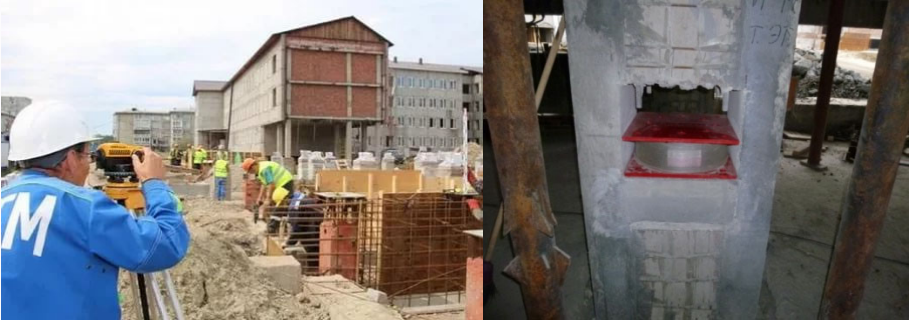
Figure 16 School building in Angarsk. Re-constructed with LRB.
