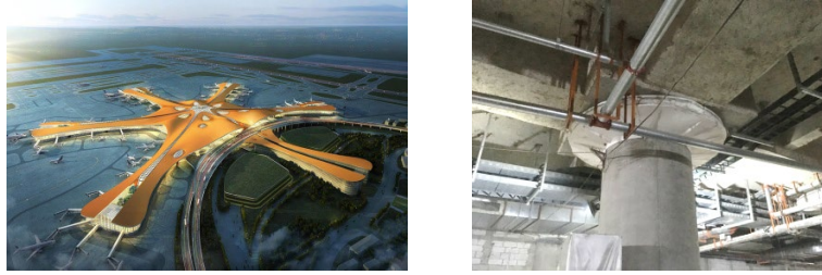
Figure 14 Seismic isolation of new Daxing airport terminal (2015-2019)
