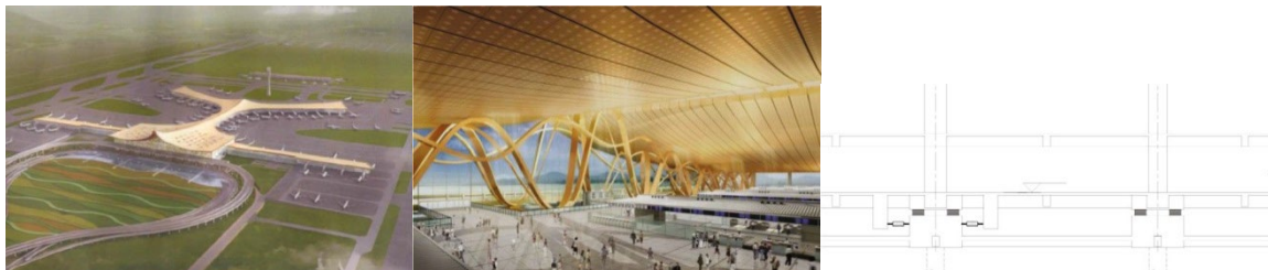
Figure 13 Seismic isolation of new Kunming airport terminal (2007-2012)
