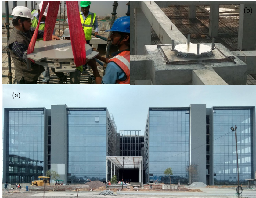
Figure 15 Photographs of the (a) Ireo Business Park, Gurugram and (b) Isolator Units and its Installation
