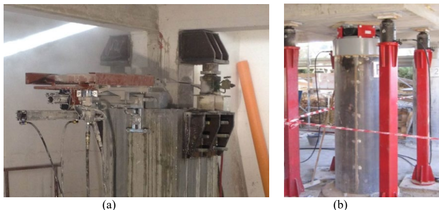
Figure 3. Typical insertion of the devices along a column: (a) cutting of the column (courtesy FIP Industriale); (b) temporary structure to unload an entire column (courtesy G&P Intech).
