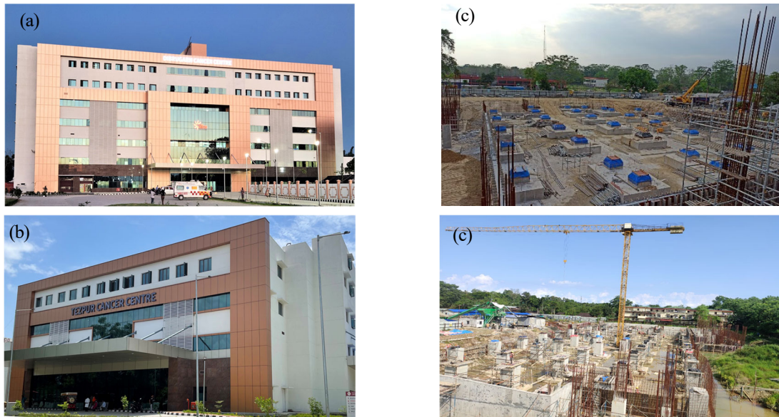
Figure 14 Photographs of the Hospital Structures at (a) Dibrugarh, (b) Tezpur, and (c) During Construction Images
