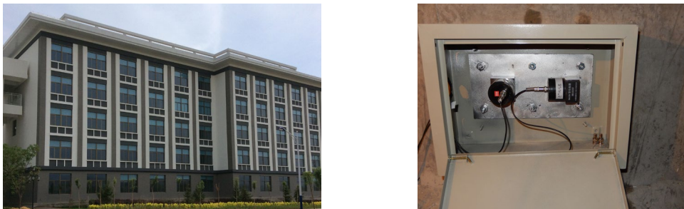
Figure 31 Acceleration sensor layout of a school building (Du et al. 2018)
