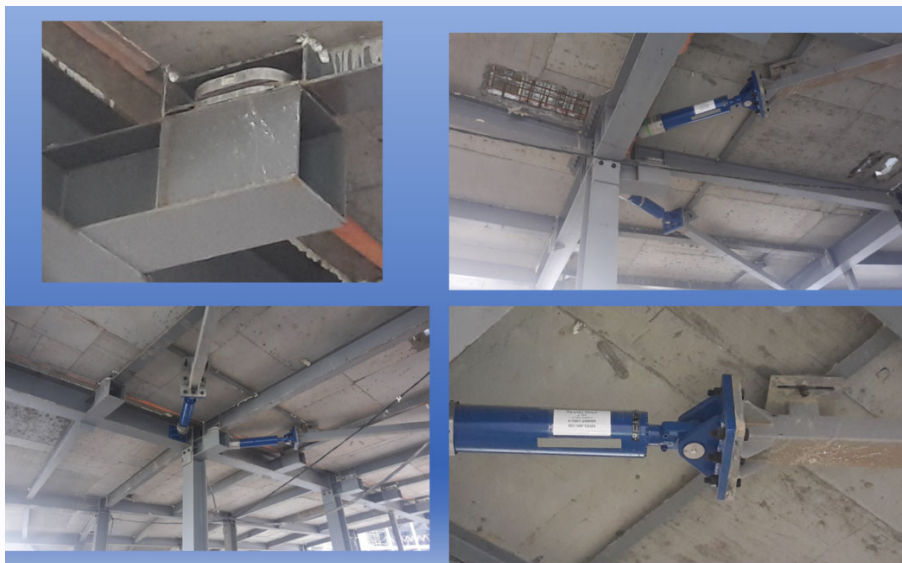
Figure 15 School building in Sochi (dampers and sliding supports)
