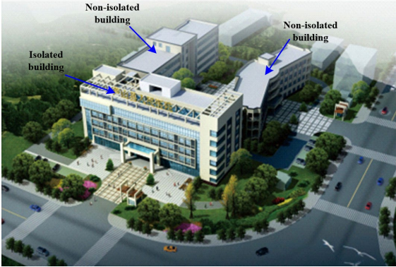
Figure 1 Lushan County Hospital, including three buildings
