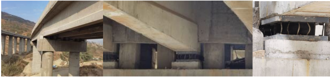
Figure 19 Datianba #2 highway bridge with SMA-HDRs in Yunnan Province, China
