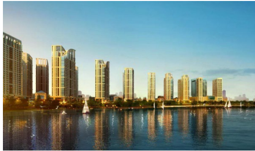
Figure 10 Seismically isolated residential apartment buildings
