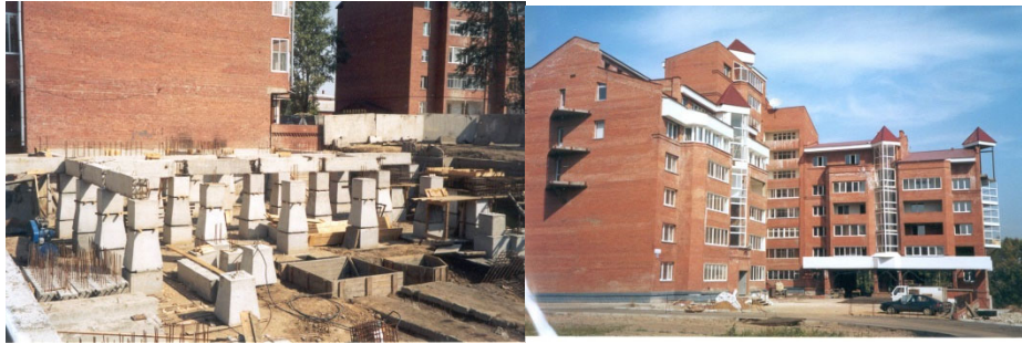
Figure 4 Buildings on kinematic supports in Irkutsk
