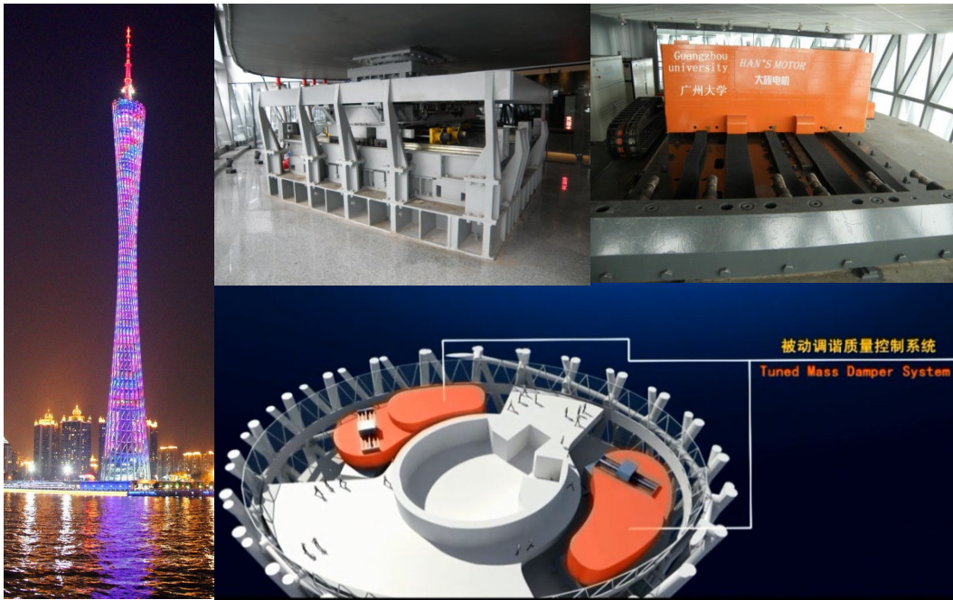
Figure 28 Hybrid control system consisting of two water tanks as TMD and two AMDs for Canton Tower
