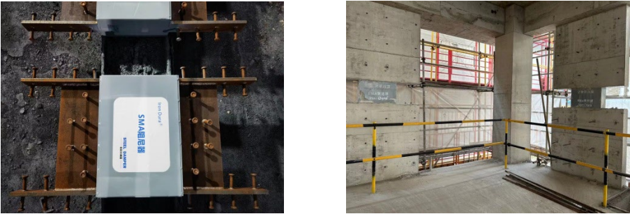
Figure 26 New Fe-SMA shear damper for shear wall structures
