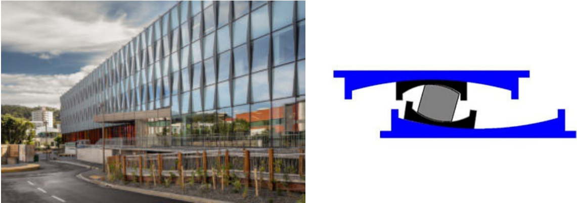
Figure 2. Left: New isolated Wellington Children's Hospital. Right: Triple Pendulum™ isolator diagrammatic.
