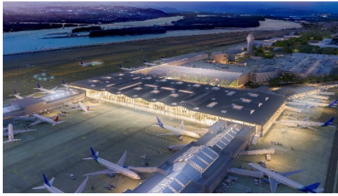
(a) Exterior view, main terminal building
