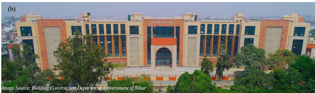
Figure 5 (a) Structural Framing Showing Isolation Level and (b) Pictorial View of the Sardar Patel Bhavan, Patna, Bihar
