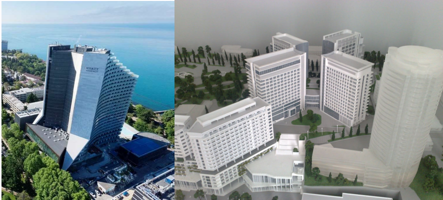
Figure 9 Seismic isolated high rise Hotel (left) and Olympic university (right) in Sochi
