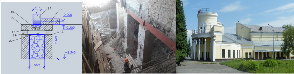
Figure 11 Seismic isolated building of Communar Theatre in Novokuznetsk city (left) and in process (middle)
